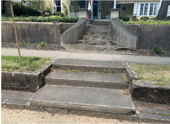
Stairs and portion of L & R wall
