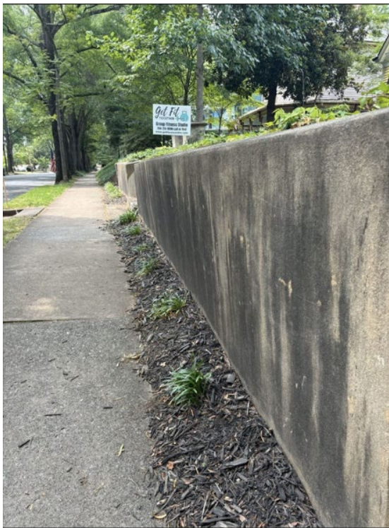
Wall facing North (right side nearest)
